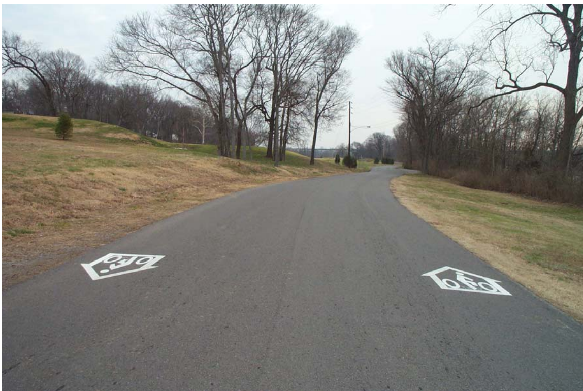
Figure 24: Pavement markings for wide outside lanes
