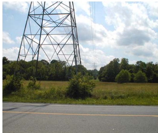
TVA Electric Power Corridor
