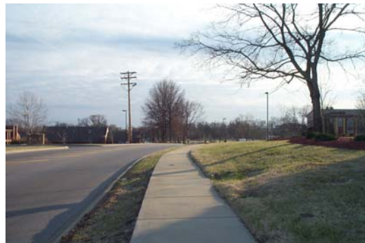
Sidewalk in Good Condition
