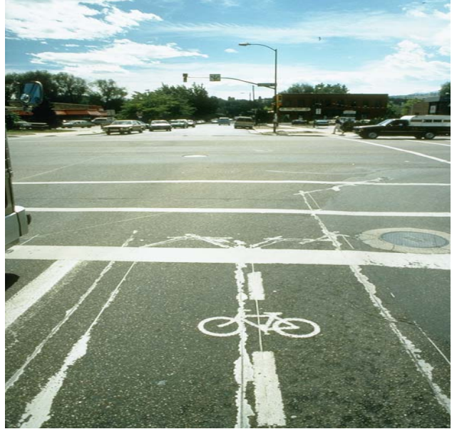
Figure 16: Pavement marking to indicate location of detector loops
